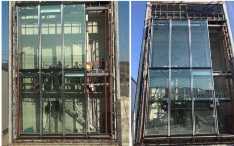
Figure 4. Full Scale Mock-up Test [17]
