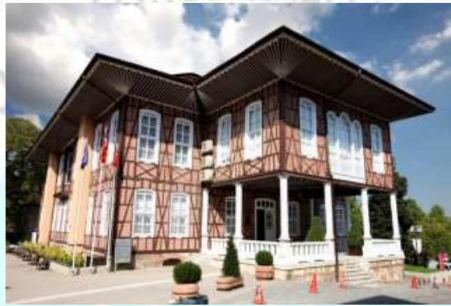
Fig. 2. Traditional himis building with bracing elements and brick infill in Bursa
