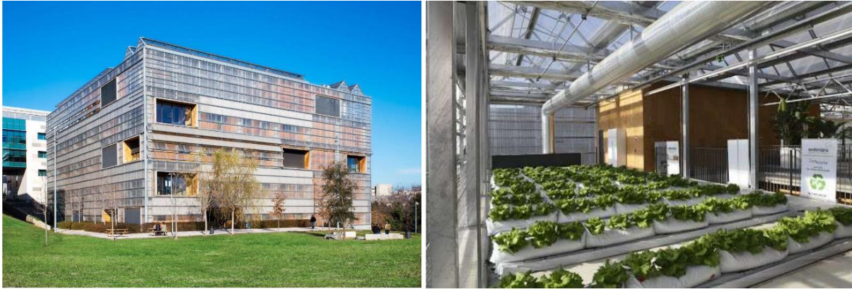
Visual 6. View from an example of a rooftop greenhouse [28]
